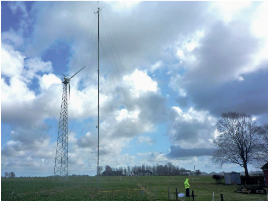
Figure 11: A WindEn 45 turbine undergoes testing by Intertek
